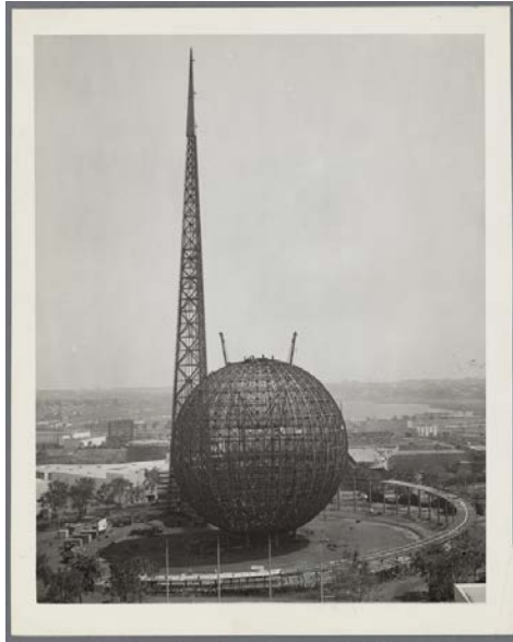
Figure 32. Steel framework of Trylon and Perisphere.
